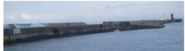
Fig.17 The caissons of offshore breakwater in Fushiki-Toyama Port were moved a few meters to 12 meters by swells which were invaded Toyama Bay on February 24, 2008
